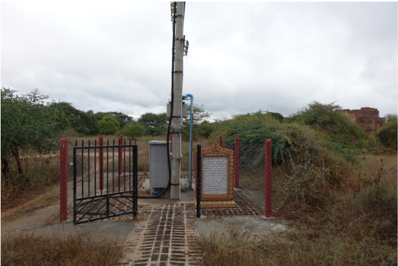
Cell tower in Bagan, central Myanmar. Credit: author.
