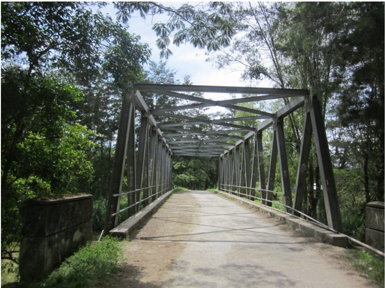
Road and bridge in Jayawijaya, Papua, Indonesia. © 2020 Jacob Nerenberg
