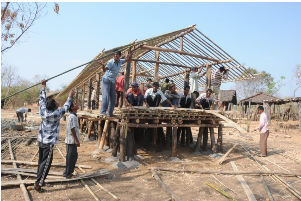
Fig. 1 Tribal Habitat under construction by tribal artisans at the Indira Gandhi Rashtriya Manav Sangrahalaya (IGRMS), Bhopal, showing the collaborative reconstruction of life-size tribal dwellings using traditional materials and indigenous building techniques. Source/Copyright: Courtesy of Indira Gandhi Rashtriya Manav Sangrahalaya (IGRMS), Bhopal.
