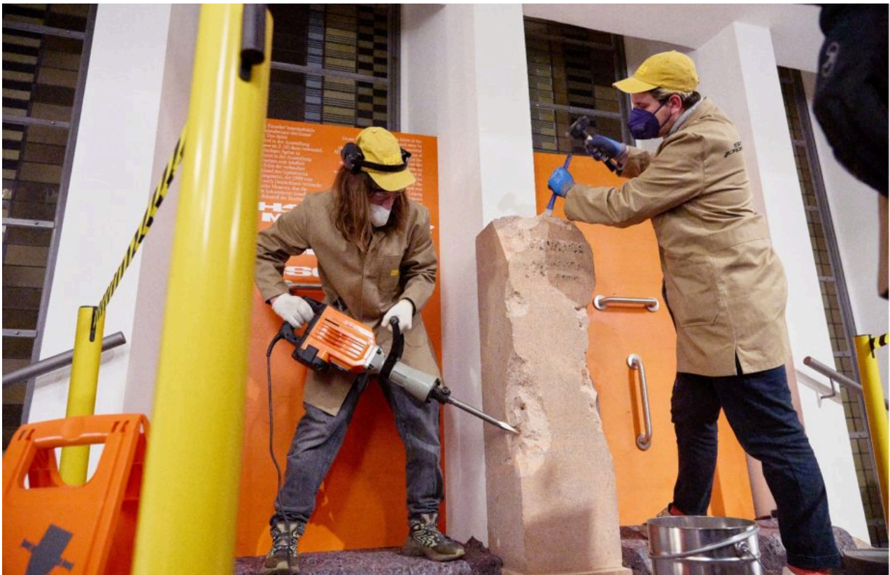
The processing of the stone pedestal on the opening evening, March 3, 2022. © GRASSI
